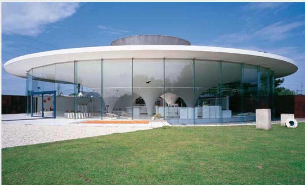
Roth radiant heating system, Keramion Ceramic Museum, Frechen, Germany
