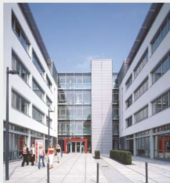
Roth Isocore®, Büro Campus Deutz office buildings, Cologne, Germany
