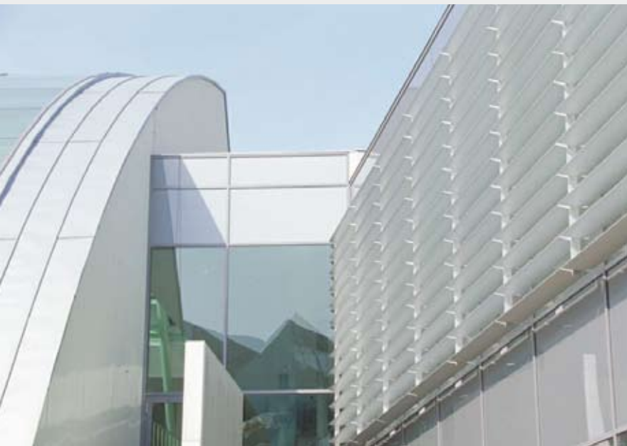
Roth radiant heating system, Niederösterreichisches Landesmuseum (Museum of Lower Austria), St. Pölten, Austria
