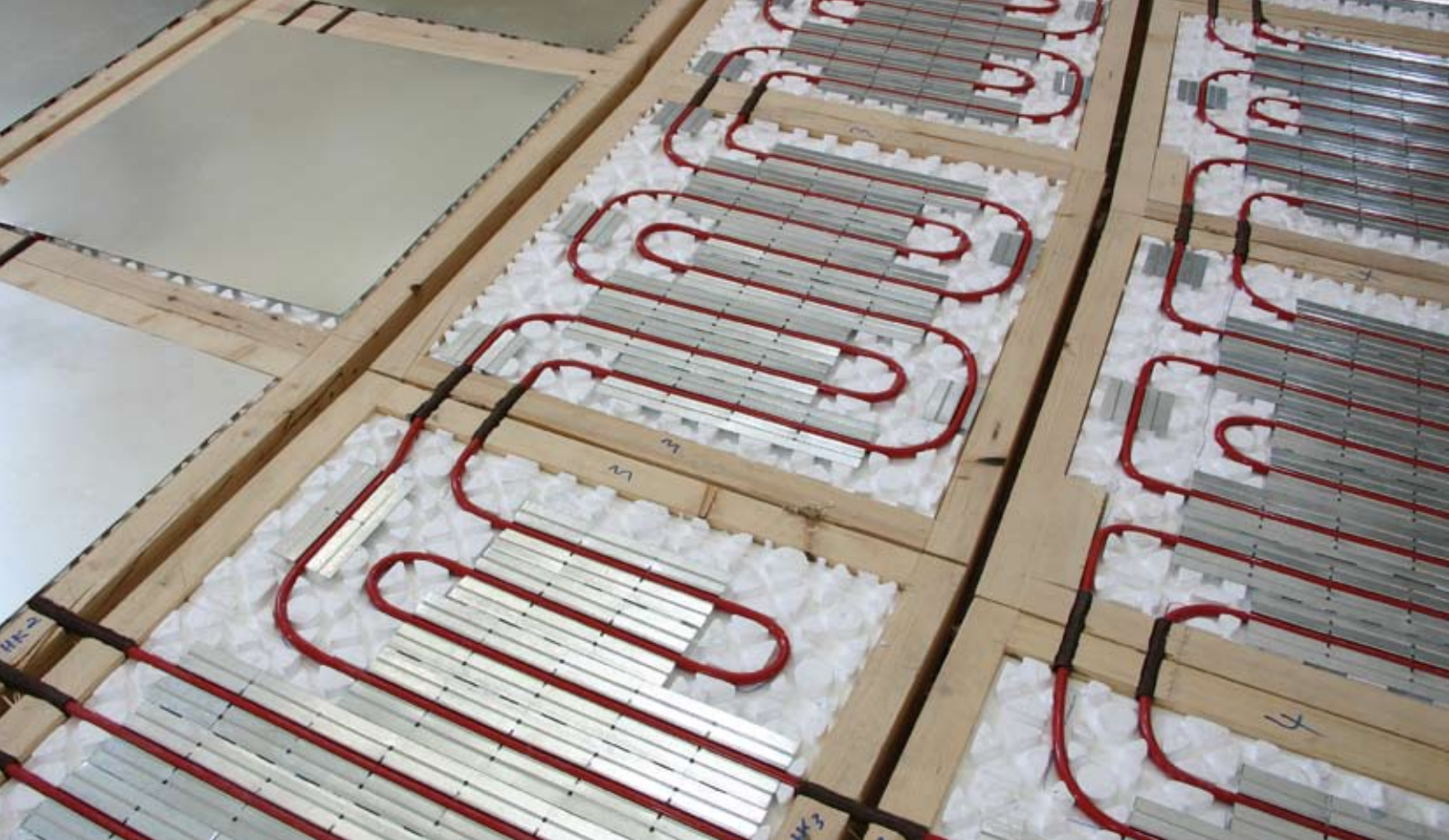
Roth ClimaComfort® DCS, Frauenkirche, Dresden, Germany
