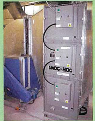
SMOG-HOG Electrostatic Precipitator installed at Miu Fat Buddhist Monastery 妙法寺內的靜電除油煙器
